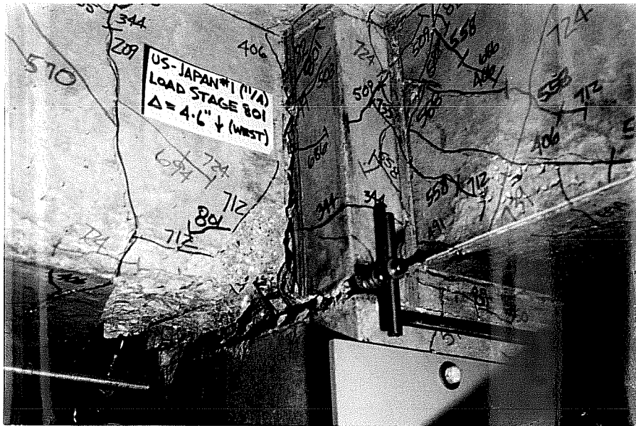
Fig. 4.25 Cracking near NE corner of joint, Test 5
