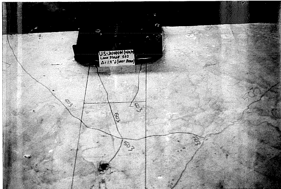
Fig. 4.18 Cracking in slab near loading points
